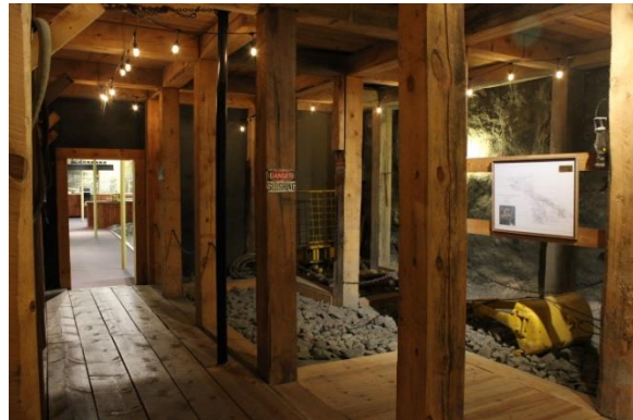
Figure 3 Replica Square Set Timber Stope
